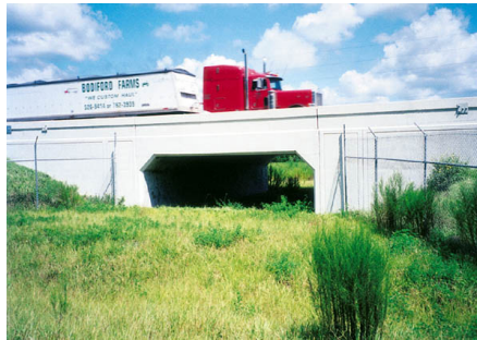
Florida State Route 46 was elevated over this underpass. Notice the channeling fences on either side of the crossing.
